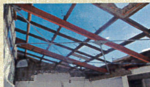
Renforcement de charpente
